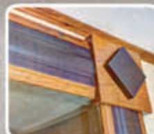
CROWN MOLDING IN LIVING ROOM
